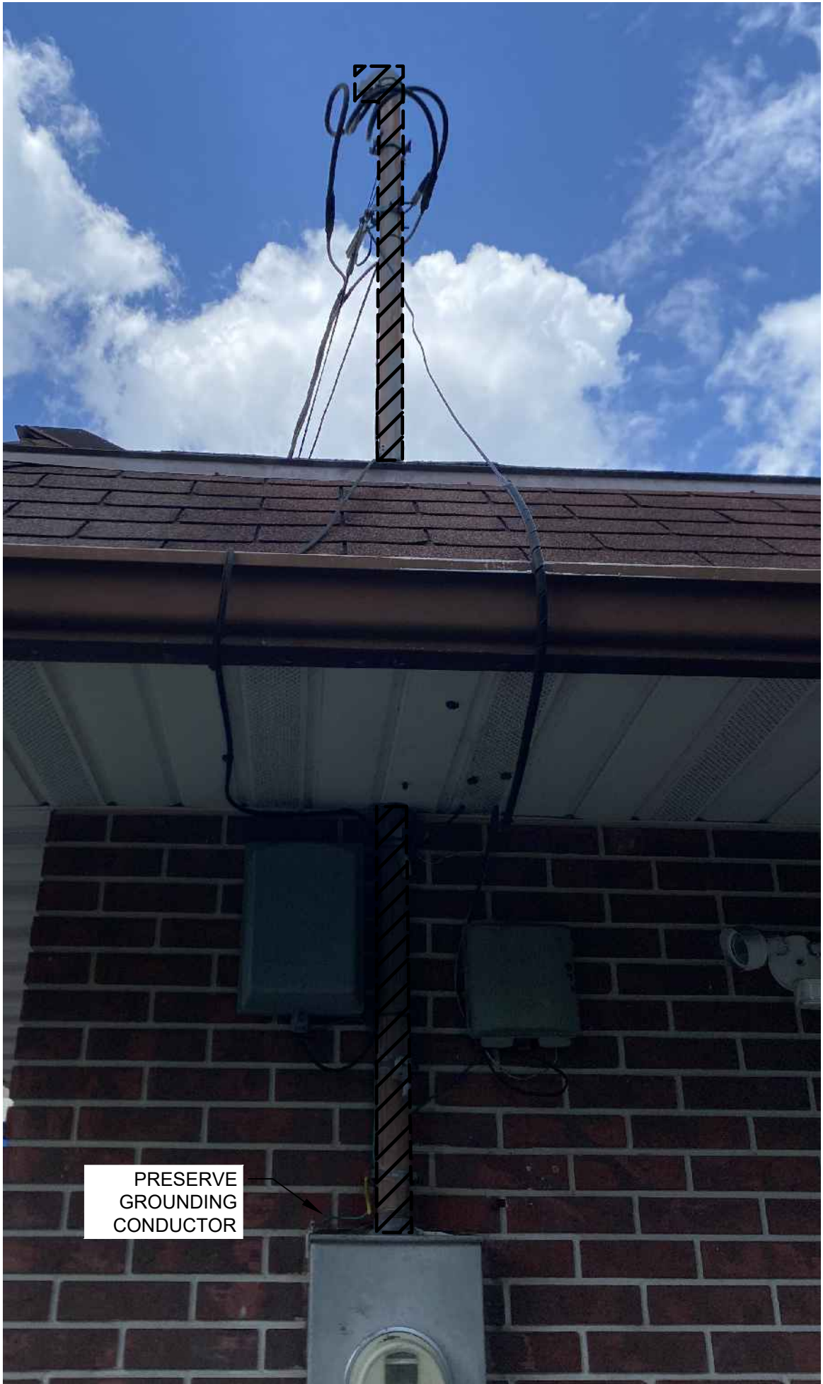
1 1349 RIDGEWOOD AVE POWER PLAN - DEMOLITION
