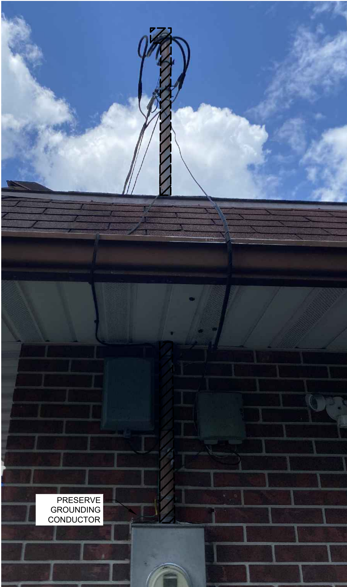
1 1349 RIDGEWOOD AVE POWER PLAN - DEMOLITION
