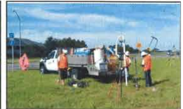
Subsurface Utility: Designation/Location
