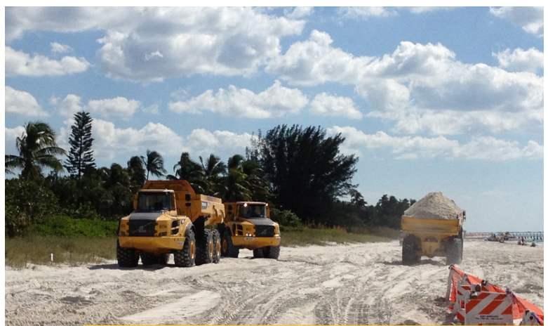
2013 Collier County, FL Beach Renourishment
