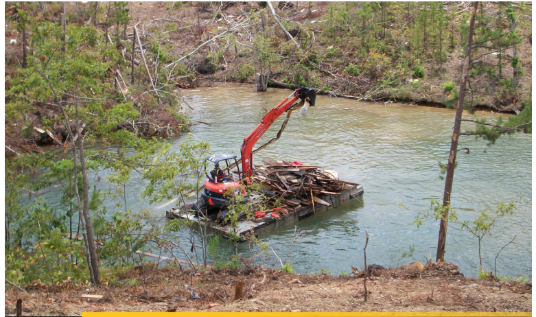
2011 AL Tornado Super-Outbreak Marine Debris Removal
