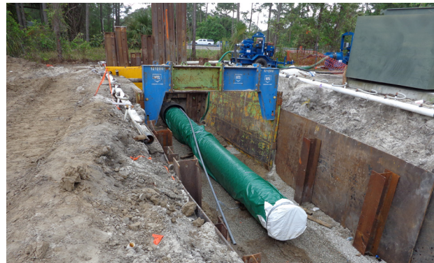
McKim & Creed, as engineer of record for Daytona Beach, completed this jack and bore under Interstate 95.
