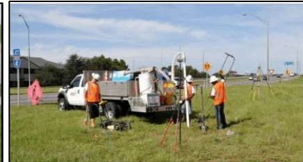
Sub-Surface Utility Designation/Location
