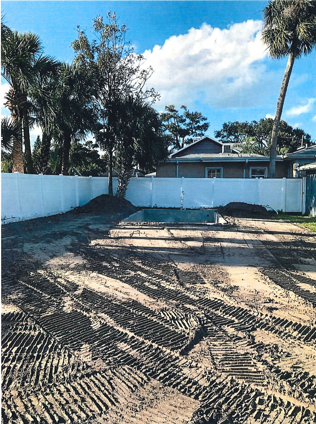
View to North rear property line towards parcel #0041
