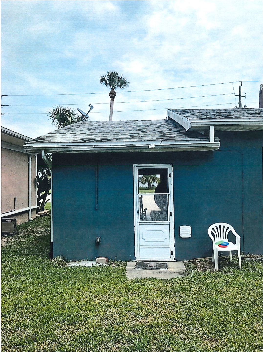
Existing condition at north property line towards Parcel #0041
